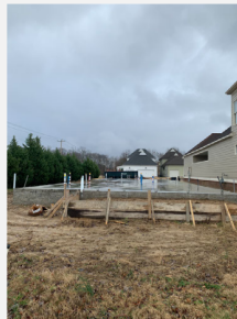
Construction slab at the end of Magilbra
